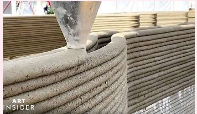
Figure 4: 3D Printed Building Structure
