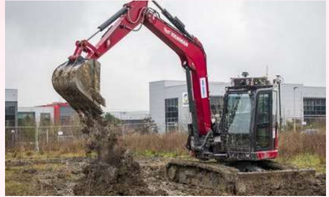
Figure 3: Autonomous Excavator in Construction Site
