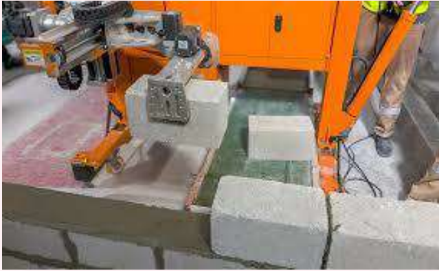
Figure 1: Robotic Bricklaying in Construction Engineering
