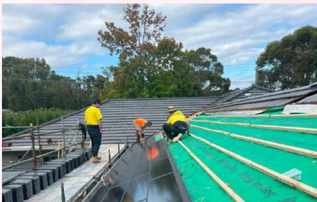
Fig 3: Solar panel roof installation
